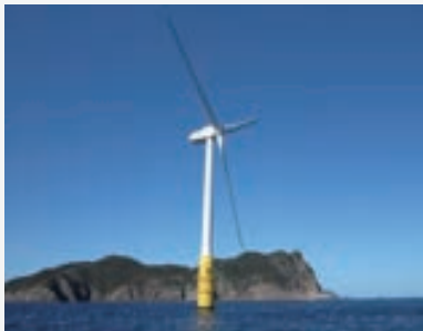
2-MW spar-type floating wind turbine
