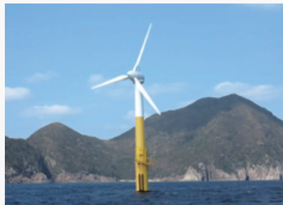
1/2 model of 2-MW real turbine in actual sea area demonstration test
