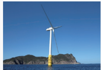
2-MW spar-type floating wind turbine
